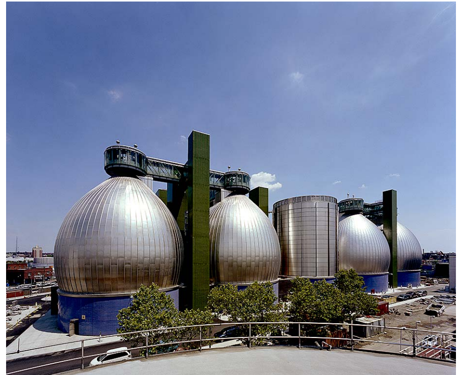
Newtown Creek waste water treatment plant in Brooklyn, NY
