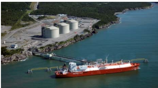
Canaport LNG. Photo courtesy of Repsol
