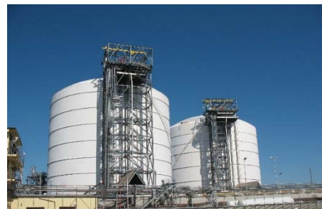
Everett LNG facility, part of Exelon (Constellation)
