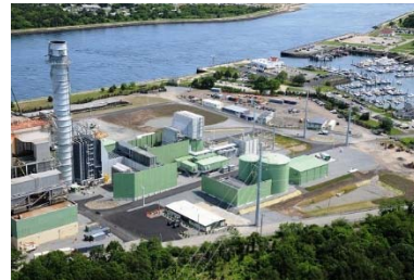
NRG Canal 3 Sandwich, MA 333 MWs Online June 2019
