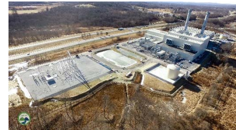
CPV Valley Energy Center Center Wawayanda, NY 680 MWs Online Fall 2018
