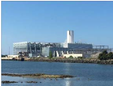
Footprint Power Salem Harbor Salem, MA 674 MWs Online June 2018
