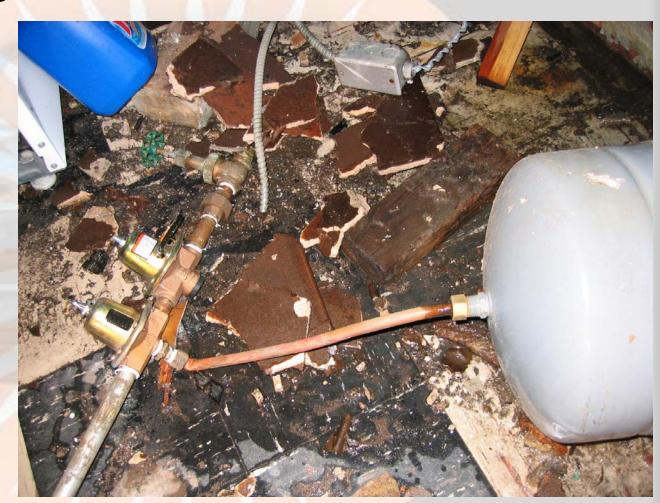
The explosion launched boiler sections throughout the basement.
