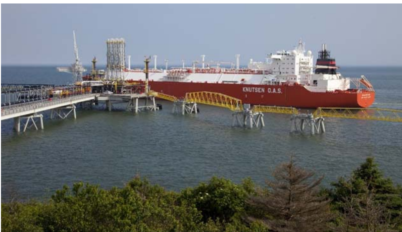
LNG ship making delivery at Canaport facility, June 2009 (photo: Canaport LNG)
