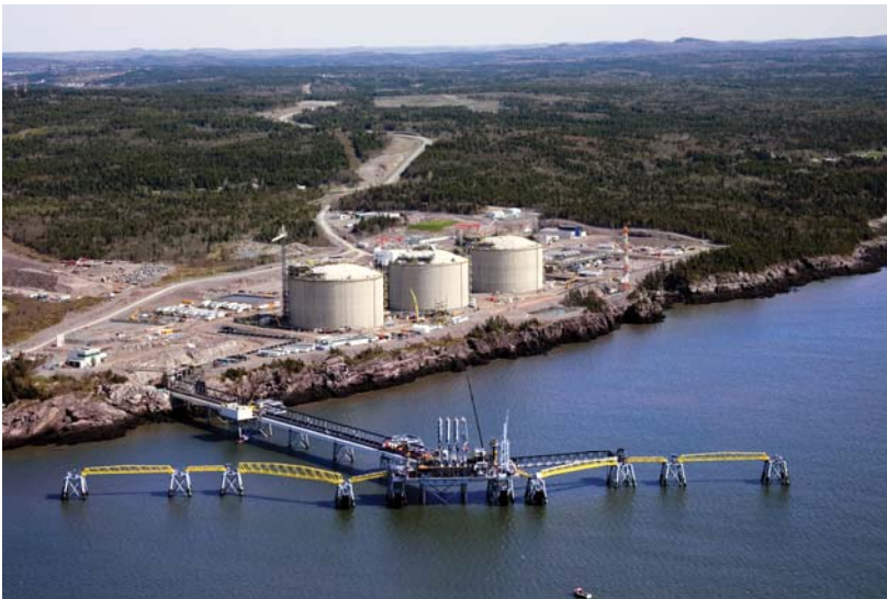
Canaport LNG facility, New Brunswick, Canada (photo: Repsol)
