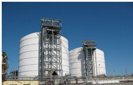
Everett LNG facility, part of Exelon (Constellation)
