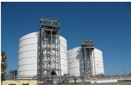
Everett LNG facility, part of Exelon (Constellation)
