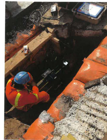
Figure 2: Field installation of a 12" BFRS on a HDPE low-pressure gas pipeline.
