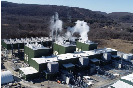
Photo: Cricket Valley Energy Center
