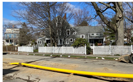
A natural gas distribution line being up-graded and about to be installed, outside Boston, in spring 2021.
