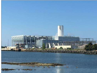
Footprint Power Salem Harbor Salem, MA 674 MWs Online June 2018
