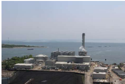
PSEG Power Bridgeport Harbor Station 5 Bridgeport, CT 485 MWs Online June 2019
