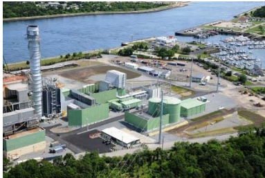
NRG Canal 3 Sandwich, MA 333 MWs Online June 2019
