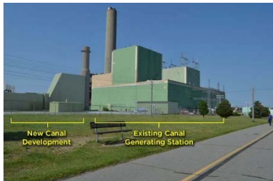
NRG Energy Canal 3 Sandwich, MA 333 MWs Single-cycle peaker Expected online, June 2019
